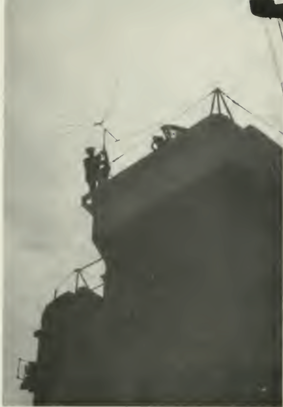
LEFT: AN RCA TECHNICIAN, WORKING HIGH ON THE SUPERSTRUCTURE, ERECTS A TELEVISION ANTENNA FOR ONE OF THE TV RECEIVERS ABOARD A CANADIAN CARRIER.
