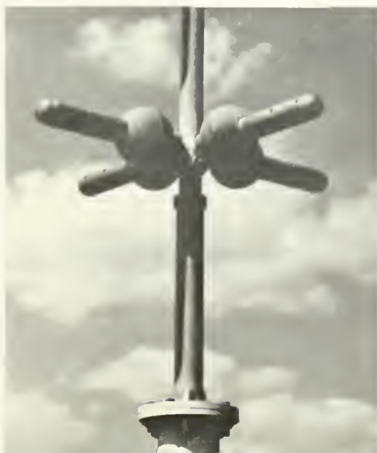
1939—THE RADIATOR PICTURED BELOW WAS ONE OF THE UHF UNITS ADDED TO THE MAIN ANTENNA STRUCTURE FOR EXPERIMENTAL USE.
