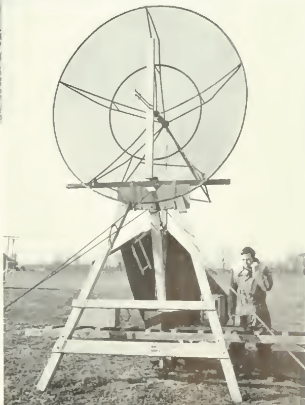
PARABOLIC RECEIVING ANTENNA BEING TESTED BEFORE INSTALLATION ON THE STATION'S TOWER.
