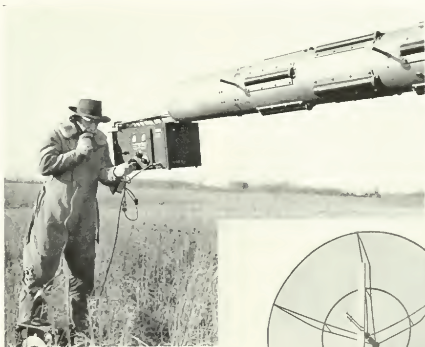
ENGINEER TUNES SLOT-TYPE ANTENNA BEFORE IT IS LIFTED TO TOP OF 210-FOOT TOWER OF BRIDGEPORT STATION.
