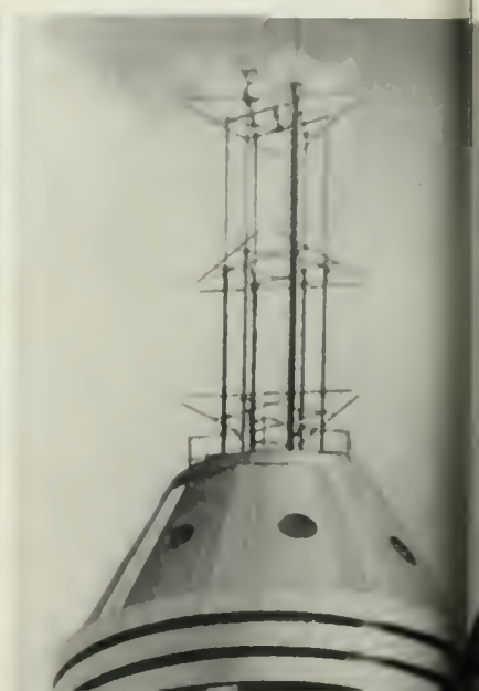
1936—AN ARRANGEMENT OF POLES AND RODS SUPPORTED THE THREE TRIANGULAR ANTENNAS OF THE SECOND STRUCTURE TO BE BUILT.
