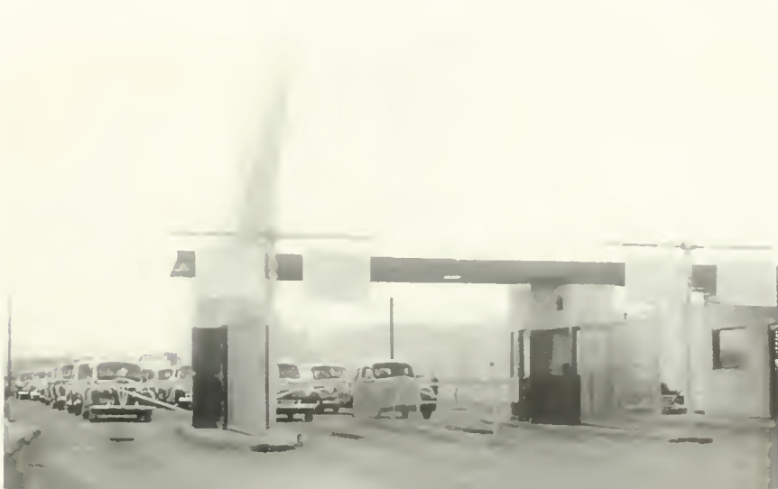
CARS MOVE UP TO TICKET BOOTH OF NEW WHITESTONE BRIDGE DRIVE-IN, NEW YORK'S LATEST OUTDOOR THEATRE. SIDE OF HUGE SCREEN SHOWS IN BACKGROUND.
