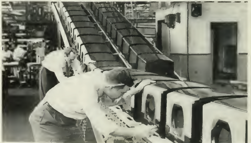
CABINETS FOR TABLE MODELS OF TELEVISION RECEIVERS (ABOVE) MOVE IN A CONTINUOUS LINE AT RCA'S CAMDEN PLANT, WHILE COMPLETED 16-INCH TELEVISION CONSOLES (BELOW) RECEIVE FINAL ADJUSTMENTS AT THE COMPANY'S INDIANAPOLIS FACTORY.
