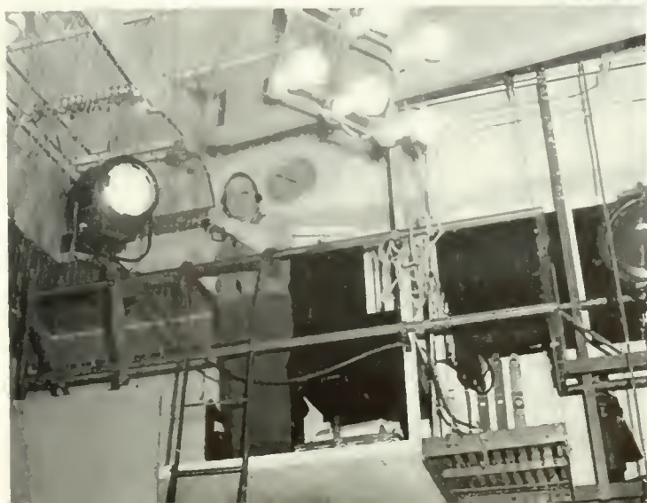
7 Stage illumination is controlled by a network of cables operated from this lofty gallery above the studio.
