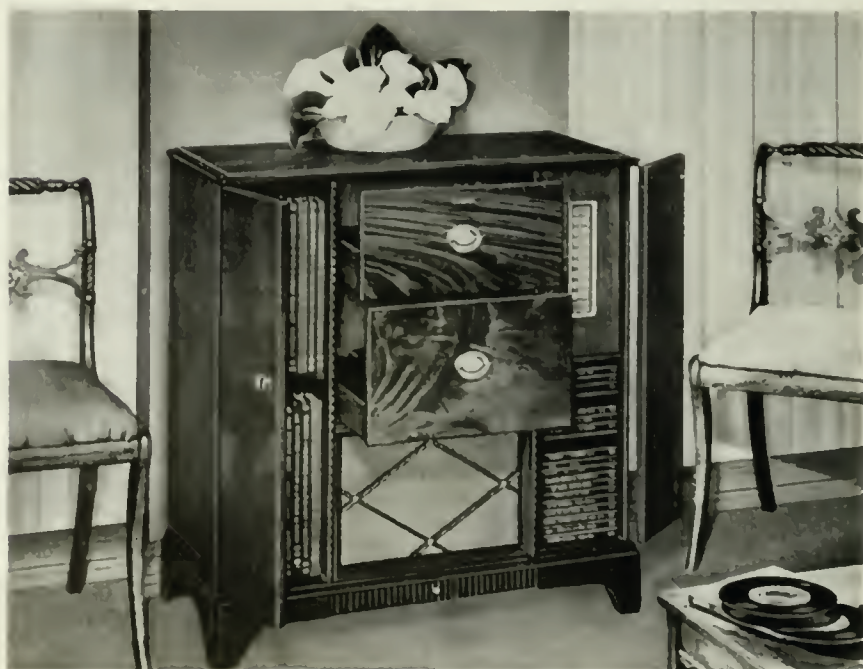
ONE OF THE NEW RCA VICTOR MODELS HAS FACILITIES FOR PLAYING BOTH 78-RPM AND 45-RPM RECORDS, IN ADDITION TO FM AND AM RECEPTION.
