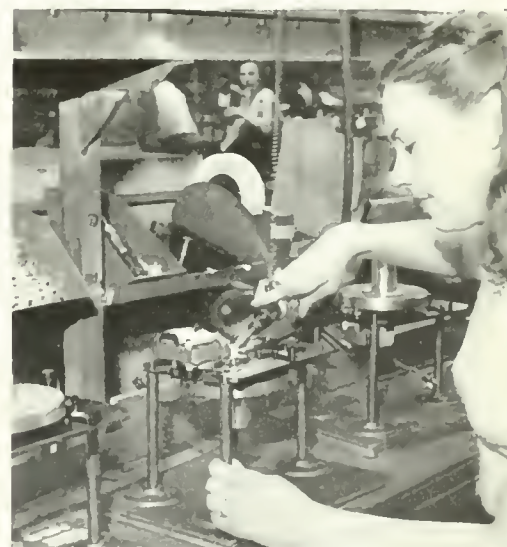
Assembling one of the basic components of the trouble-free automatic changing mechanism of the 45-rpm record player.
