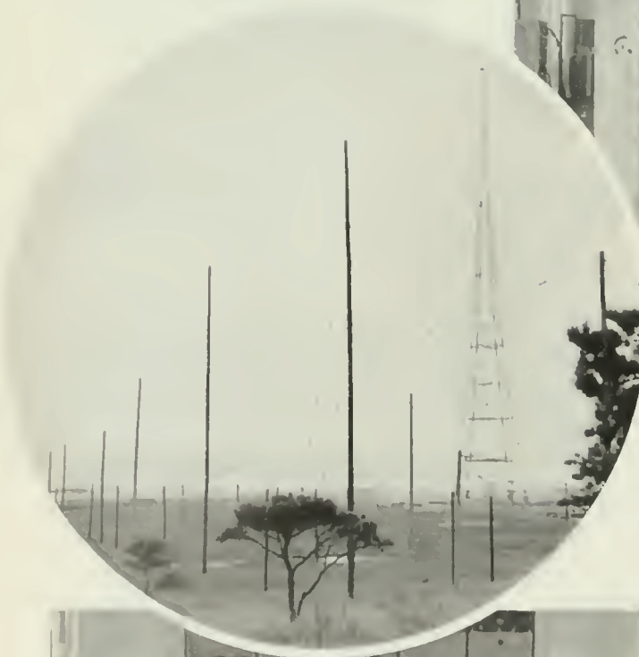
Beyond the lines of short masts supporting the station's high-frequency antennas is the high tower of Chatham's 500-kilocycle transmitter.
