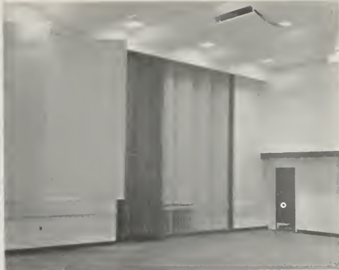
VIEWS OF NBC STUDIO 3A SHOWING UNEVEN WALL SURFACES WHICH CAN BE ADJUSTED TO CONTROL ECHOES.
