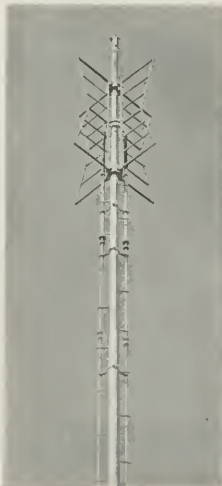
LEFT TO RIGHT: NEWLY DESIGNED SUPER-FM ANTENNA FOR FREQUENCY MODULATION STATIONS; AN EMPLOYEE EXAMINES PRESSING OF AN RCA VICTOR NON-BREAKABLE RECORD; SCIENTISTS IN RCA LABORATORIES CONSTANTLY EXTEND THE SCOPE OF RESEARCH IN RADIO AND ELECTRONICS.
