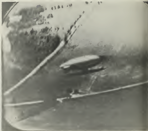
BELOW: ENGINEERS MONITOR THE INCOMING SIGNALS AS THEY ARE PICKED UP FROM NAVY AND RCA PLANES DEMONSTRATING "RING" AND "BLOCK" AIRBORNE TELEVISION SYSTEMS IN THE AIR OVER WASHINGTON AND BALTIMORE. RIGHT: ACTUAL PHOTOGRAPH OF TELEVISION IMAGE TRANSMITTED BY "BLOCK"-EQUIPPED PLANE FLYING OVER SOLOMON ISLANDS, MD., AT AN ALTITUDE OF 1,000 FEET.
