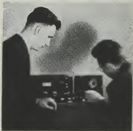
The RCA Radio Altimeter assures that the last mountains have been passed before letting down to the airport in the valley below.
