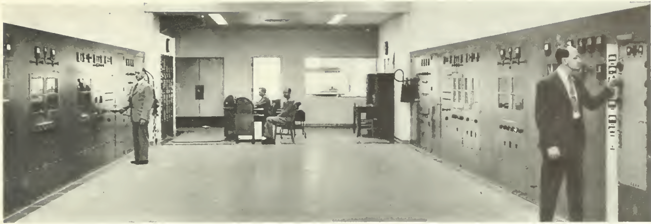
TRANSMITTER PANELS LINE BOTH SIDES OF THE CONTROL ROOM OF THE SHORT-WAVE PLANT AT DIXON, CALIFORNIA.
