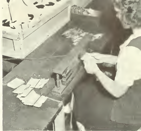
HOWEVER SMALL THE RADIO PARTS TO BE SHIPPED, THEY RECEIVE THOROUGH PROTECTION AGAINST MOISTURE-VAPOR THROUGH THE USE OF SPECIAL SEALING ADHESIVES AND CAREFUL PACKAGING.
