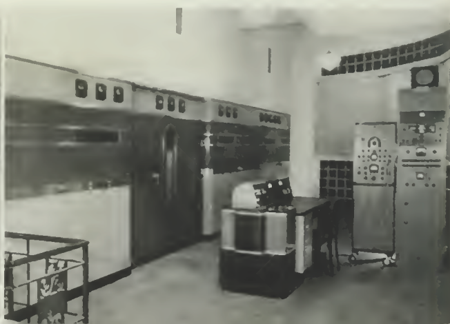
LEFT: TRANSMITTER PANELS AND CONTROL DESK AT LEOPOLDVILLE, BELGIAN CONGO. RIGHT: ANOTHER RCA 50-KILOWATT TRANSMITTER IS OPERATING FROM RIO DE JANEIRO.
