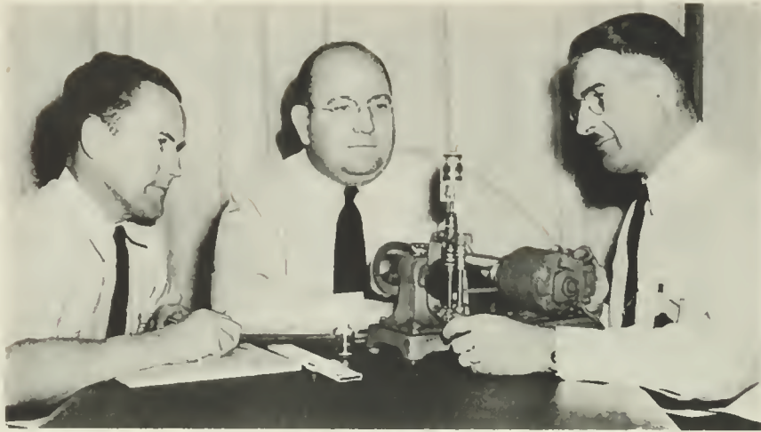
DR. GEORGE H. BROWN, INVENTOR OF THE ALL-ELECTRONIC SYSTEM FOR DEHYDRATING PENICILLIN, AND HIS ASSOCIATES, C. N. HOYLER AND R. A. RIERWIRTH, STUDY AN EXPERIMENTAL SET-UP DESIGNED TO ELIMINATE FOAMING OF PENICILLIN BROTH.
