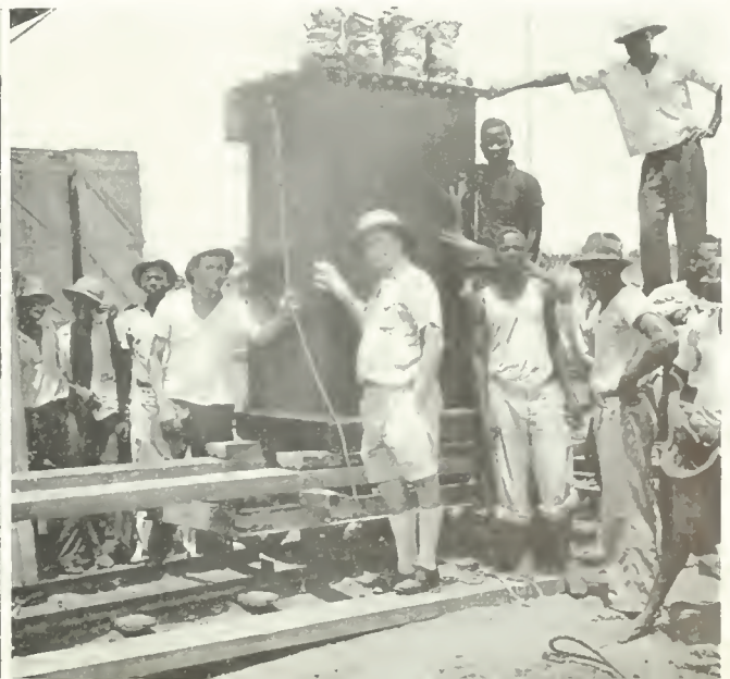
ENGINEER BROWN GETS THE HELP OF NATIVES IN PUTTING INTO POSITION THE HUGE TRANSFORMER, WHICH WAS PART OF THE RCA TRANSMITTER INSTALLATION AT BRAZZAVILLE. NO CRANES OR DERRICKS WERE AVAILABLE.
