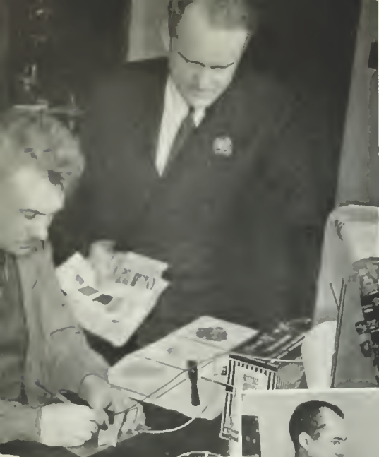
H. G. GREIG (SEATED) AND C. J. YOUNG TEST ELECTRO-CHEMICALLY PRODUCED COLORS FOR USE WITH RADIO FACSIMILE EQUIPMENT AT PRINCETON.
