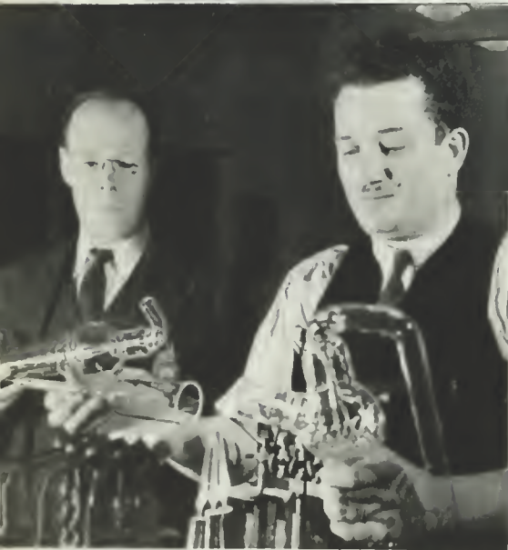
DR. R. R. LAW (LEFT) AND J. E. MC COOL PREPARE THE GLASS PARTS OF A HIGH-SPEED MERCURY PUMP FOR USE IN WORKING OUT A RESEARCH PROBLEM.
