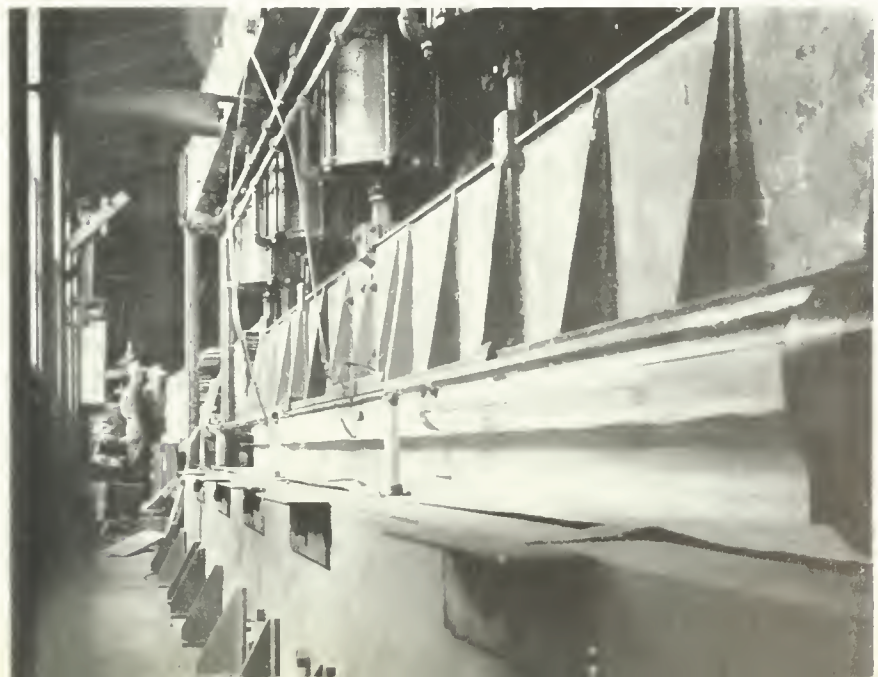
METHOD OF GLUING AIRPLANE SPARS WITH RADIO FREQUENCY SHOWN IN THIS SCENE FROM THE TOLERTON LUMBER COMPANY, ALLIANCE, OHIO.
