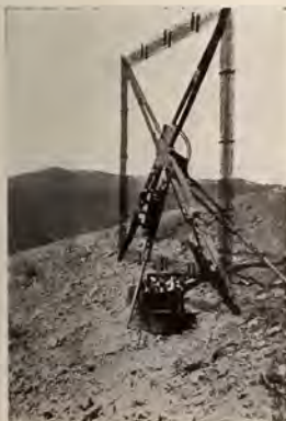
Close-up of broadcasting set which sends out alternating electric current
