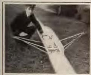
A single scull shell of duraluminum, a light but extremely durable alloy, has just been completed at the Philadelphia Naval Aircraft factory for the Annapolis Naval Academy. The shell weighs half as much as the cedar craft of the same type and size. It was built under the direction of Walter Hoover, noted single sculls oarsman. If the shell proves satisfactory, the Naval Academy expects to have an eight-oared shell constructed of the material. It is 26 feet long and weighs only 26 pounds. Photo shows Lieut. Calvin Bolste, shop superintendent, inspecting the duraluminum shell.
