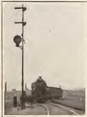
Automatic Train Stop Device is Demonstrated
