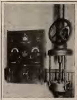
Rotation control of the radio compass loop and the receiver used for picking up directional signals.
