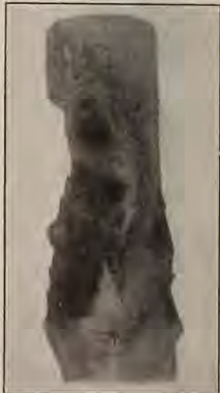
Section of tree trunk, indentation showing where wood was burned away by high power line grounding to tree
