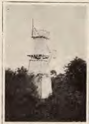
A water tank makes a convenient anchorage for the far end of the aerial, and a short mast will give additional height
