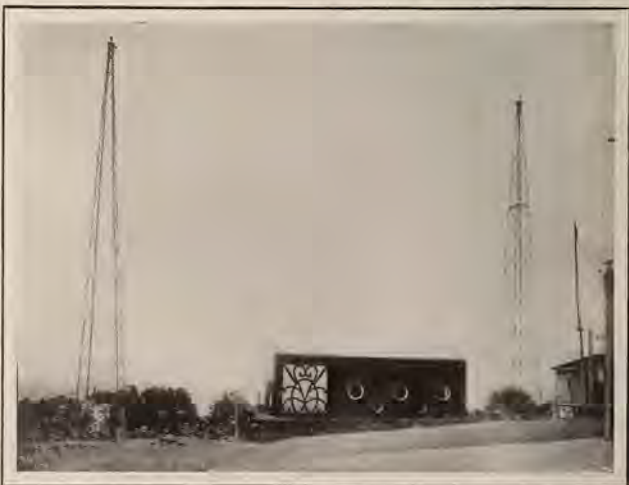
Designed to represent the Freshman Masterpiece, the studio of Station WPAP, located at the Palisades Amusement Park, New Jersey, is quite novel. The antenna is shown above the studio building
