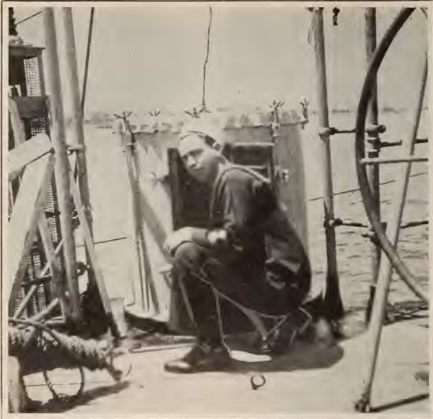
Radio compass housing mounted on upper deck. Radioman shown before the housing
