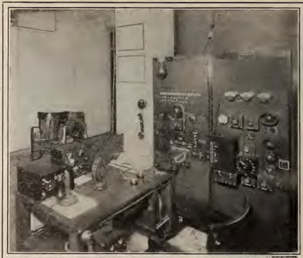
Operating Room of Station KFSD
