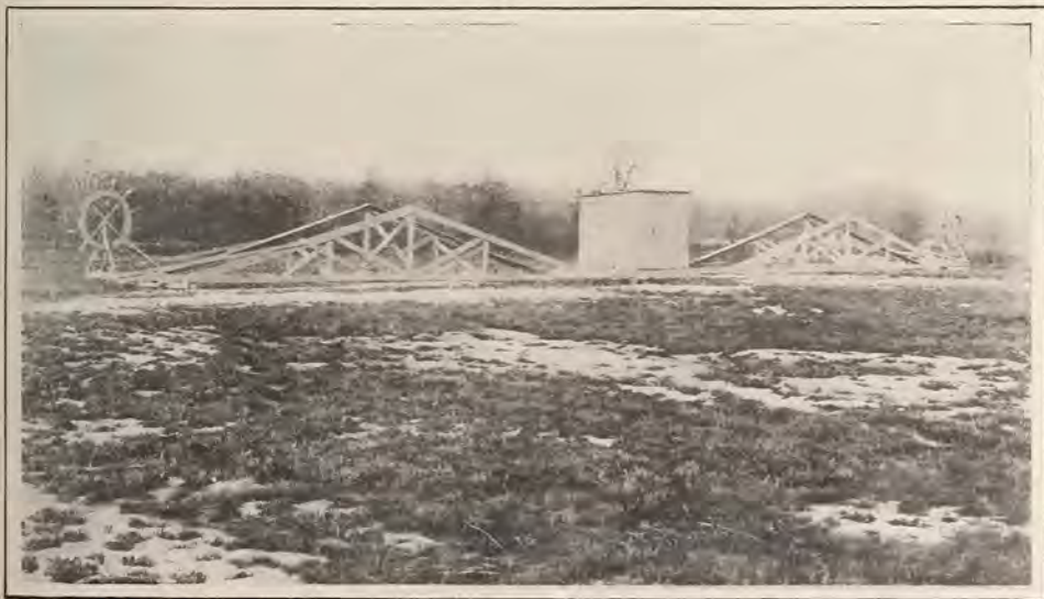
Figure 3. Two loops and receiver house where Friis' experiments were carried on
