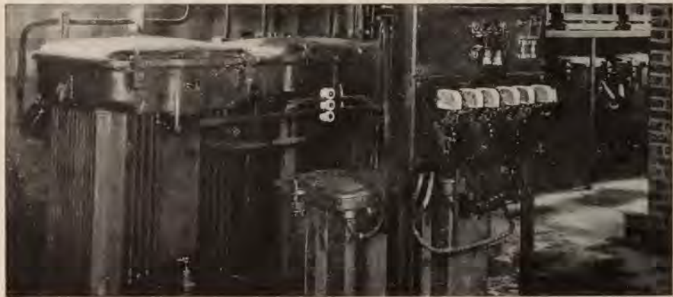
In the picture above the reader may see the amount of apparatus involved in producing the primary current necessary for a station like KDKA at East Pittsburgh, Pa., to radiate from 10 to 50 kilowatts of energy from the antenna. This enormous current at the transmitter dwindles to a few millivolts by the time it has reached your receiving antenna and must be rejuvenated in order for you to hear the signals through a loud speaker. The startling difference in size between the transmitting and receiving sets also represents the difference in the cost of transmission and reception.
