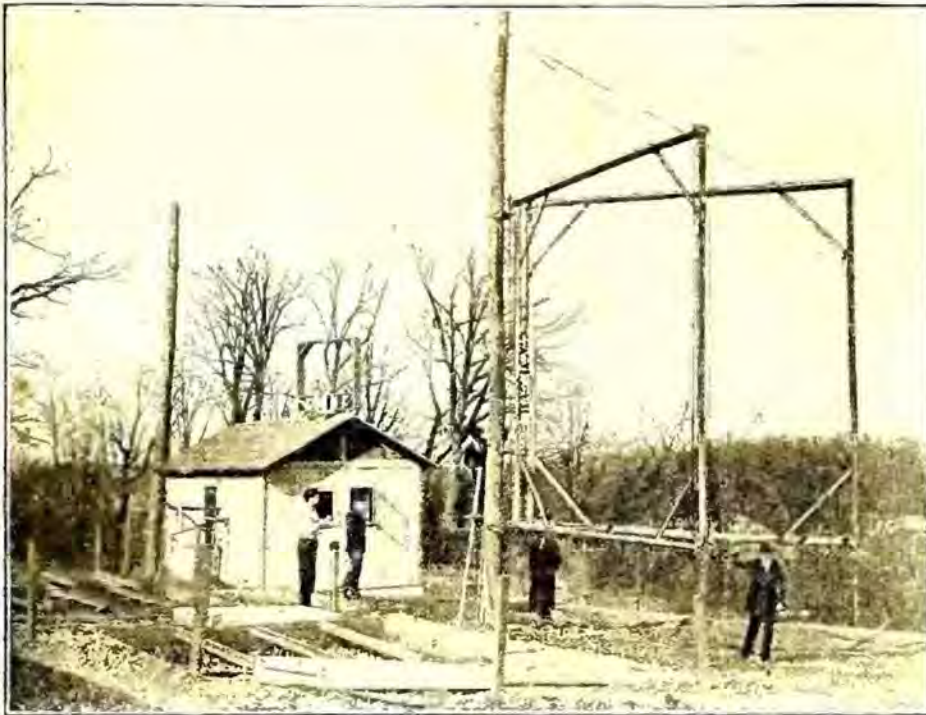
Figure 1. The photo, made by the Bureau of Standards, shows a double-coil transmitting device used for sending out radio signals whereby an airplane or ship may be guided along a straight course, thus taking the place of less reliable methods.
