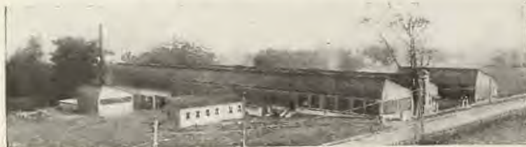
The New Liberty Electric Corp. Factory at Stamford, Conn.
