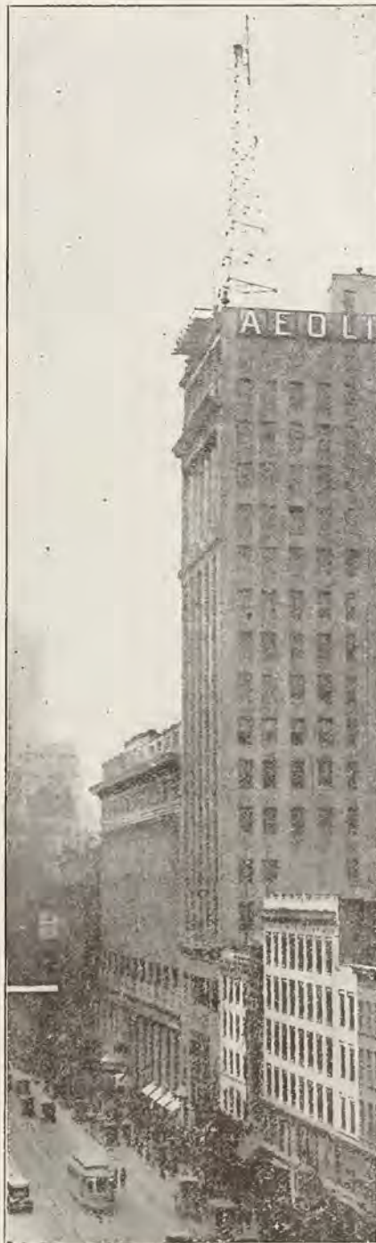
Lofty tower of the famous Station WJZ in its new home on Forty-second street, New York, between Fifth and Sixth Avenue. (U&U Foto).
