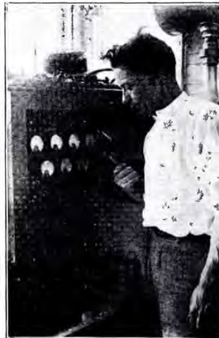
This picture shows the actual installation of the 50-watt vacuum tube transmitter on "CG198," one of the rum chasers of the U. S. Coast Guard. Both voice and telegraphic signals are transmitted with this apparatus.
