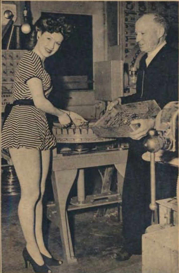
EILEEN FENWICK, 20th Century-Fox player, visits Hulbert in his shop, above, and seventy-one-year-old inventor shows her how his nail-reclaiming machine works. Below: Eileen operates the turntable that straightens the nails in grooves and turns them out ready for use again on sets
