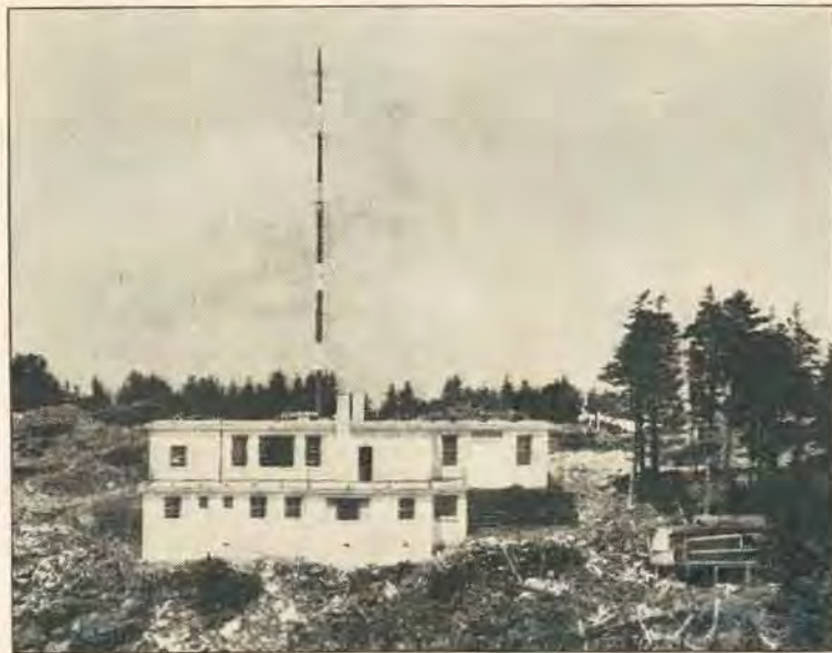
ON TOP of Clingman's Peak, 6,800 feet above sea level, sits W41MM's new transmitter building. Programs originate in W41MM's Winston-Salem studios more than one hundred miles away and are carried to transmitter for broadcast by FM radio relay. This picture was taken from an airplane
