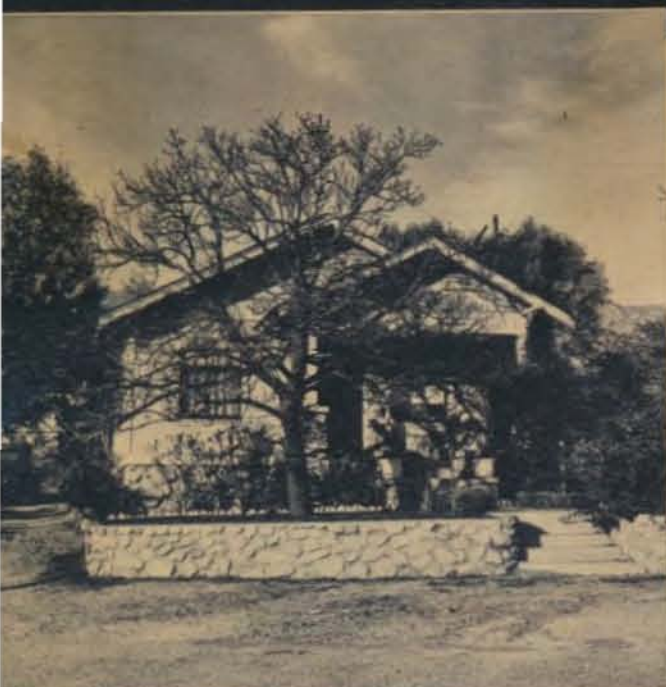
1. THIS is the house the Joe Smiths live in at La Crescenta, California. It has two bedrooms, a kitchen, bathroom and a combination living-room and dining-room. The Smiths get it, partly furnished, for thirty-two dollars a month. There's a garage and a back yard full of fruit trees
