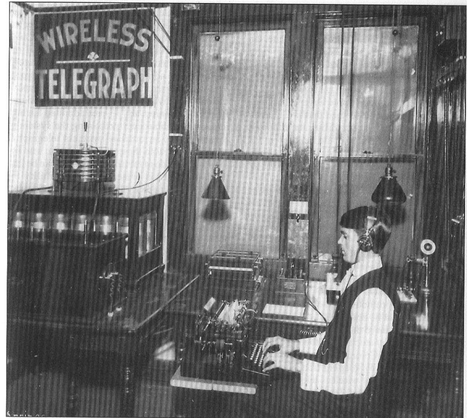
Elmo Pickerill, former AWA member and now a Silent Key, operates an American DeForest Wireless Telegraph Co. station in Colorado, 1906. Fixed-gap spark transmitter has condenser made up of 18 Leyden jars; receiver (center) is a 3-coil tuner with electrolytic detector. (Photo Courtesy AWA Museum)
